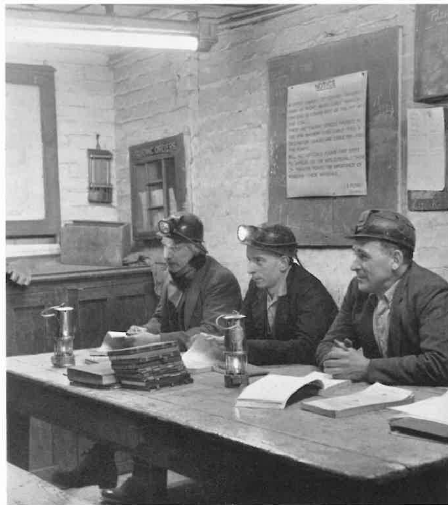
(13) In the Inspectors' Office, just off the main underground roadway at Mansfield, the same high-level of illumination is obtained. Mazda 5-ft. fluorescent fittings provide lighting comparable with that in offices above ground.
