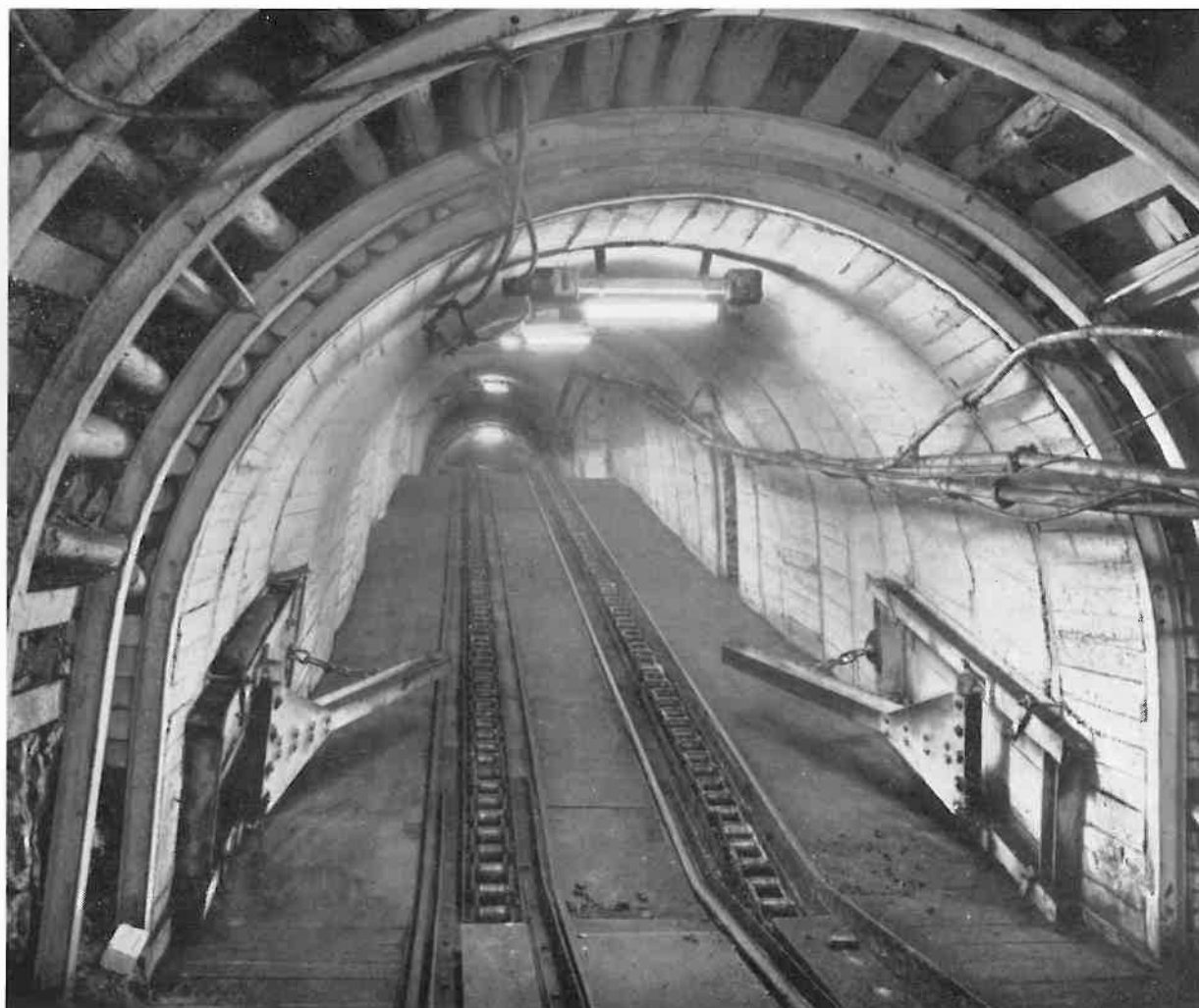
(10) With progress in mining practice, the complexity of underground roadways has increased rapidly. Interweaving haulage traffic, loading points, control rooms—all need good lighting for this safe and efficient operation. Here, the bright conditions provided by a modern fluorescent system are obvious. (11) Loaded trucks pass from the coal face to the shaft along a well-lit road to be unloaded by the fast, automatic 'tippler' seen in the foreground. (12) Fluorescent fittings stretch as far as the eye can see along another busy roadway.
